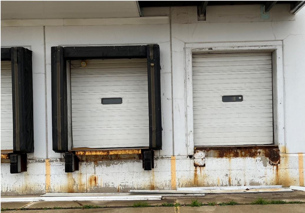
The photo above depicts what the building looks like after the sill, seal, and bumpers have been removed (threaded attachments remain as the removal was not complete). The steel, dock edge angle remains in the photo and as noted on the plans as it gets covered with metal flashing where the doors are infilled with metal panel or storefront.
